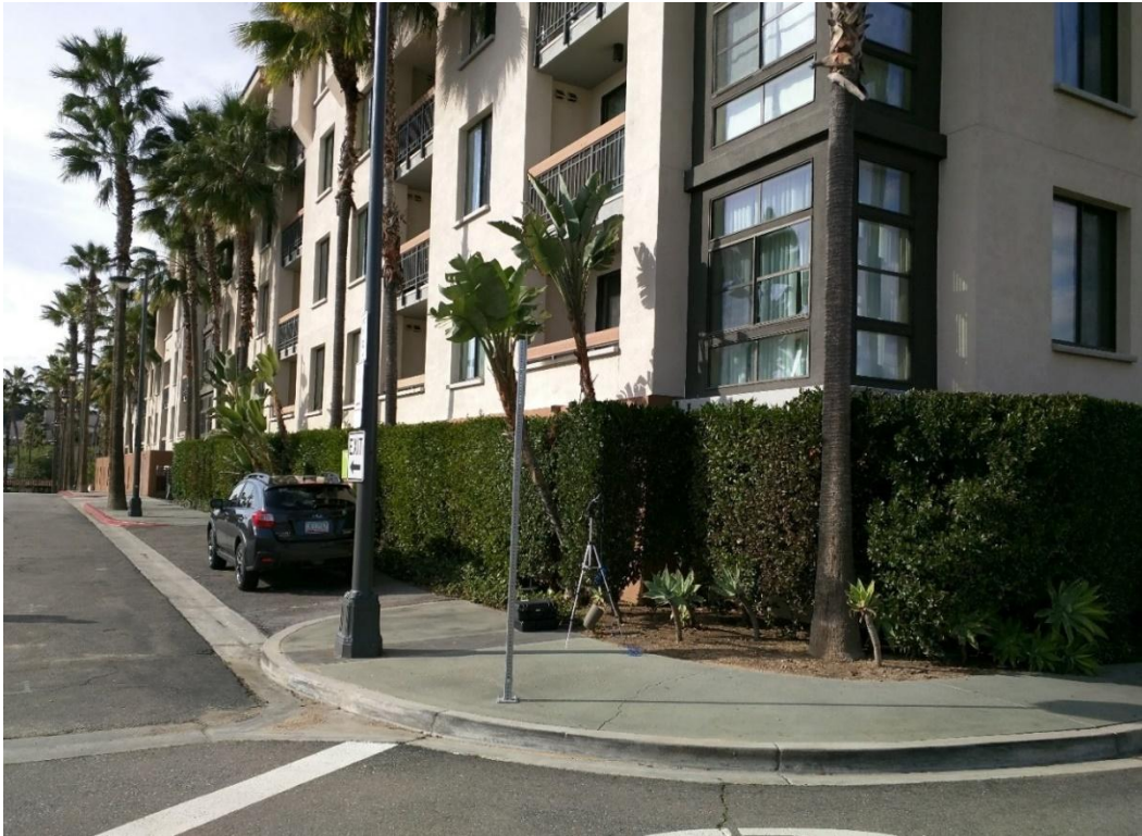
Figure 7-13. Monitoring Location 3 – Vibration Measurement at Mozaic Apartments
